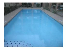
Fair condition. Chipping noted. Plaster pool. Approximate 955 SF. Acid wash was performed by Tropical Water Pool Service and Repair at end of 2015.
