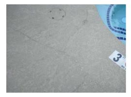
Fair to good condition. Recommend recoating due to cracking. Approximate 710 SF.
