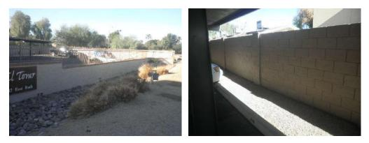
Good condition. This asset is for repairs of \$1000 every 5 years based on the condition. Approximately 840 SF - 4' high painted stucco block wall on north side, 1,470 SF - 7' high dooley wall on east side and 2,760 SF - 6' high painted stucco block wall on west and south side
