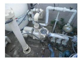
Working condition. This asset is for repair of pump and/or motor every 2 years for total \$500. Pentair Whisperflo variable speed mgf date 9/2012 - replacement cost \$1400
