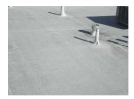
Good condition. Some chipping/peeling noted. Roof if tar based and elastomeric coated. Recommend inspection by professionals to determine if foam roof should be replaced and not just coated.
