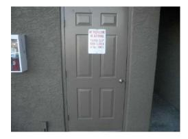
Good condition. Metal doors leading in and out of stairwells and to roof. 3.0 X 6.8. The useful life of this asset has been extended due to its present condition.
