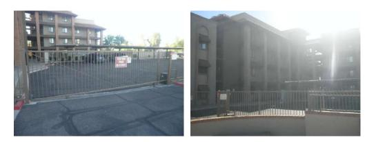
Good condition. (2) 6' X 24' sliding gates +(1) 4' pedestrian gate. The useful life of this asset has been extended due to its present condition.
