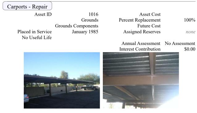
Good condition. All steel supports with corrugated metal roof. Painted support structures. Unfunded as this asset should last lifetime of condominium. Minor repairs, as needed, may be covered by the operational budget, operational contingency or insurance. Should the client feel otherwise, we will be happy to incorporate this element into our analysis.
