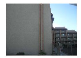
Good condition. Metal downspouts. (18) each. 1 missing.
