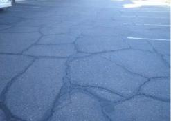
Poor condition. Recommend HA5 (high density mineral bond) for surface treatment as it does not track into condos, warranty for 5 years (lasting around 7 - 8 years) and holds color.
