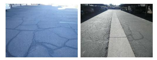
Poor condition. Recommend crack seal with slurry seal due to cracking and deterioration around valley gutter. One time asset to be followed by surface treatment the following year.
