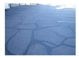
Poor condition. Recommend crack seal with slurry seal due to cracking and deterioration around valley gutter. One time asset to be followed by surface treatment the following year.
