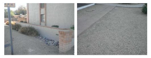
Poor condition. Recommend replenishment. This asset is approximately 10,000 SF or around 40 ton for 1.5" coverage.
